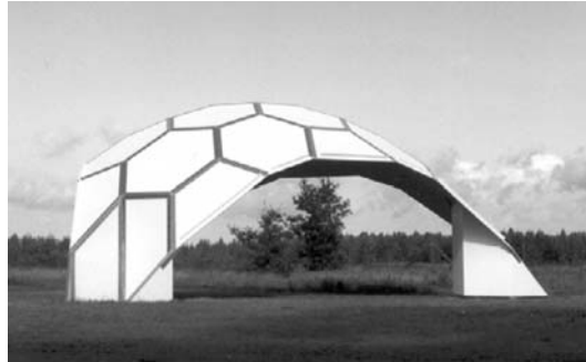
Figure 2.14: A faceted shell structure in Hørsholm, Denmark. (Almegaard 2003)
