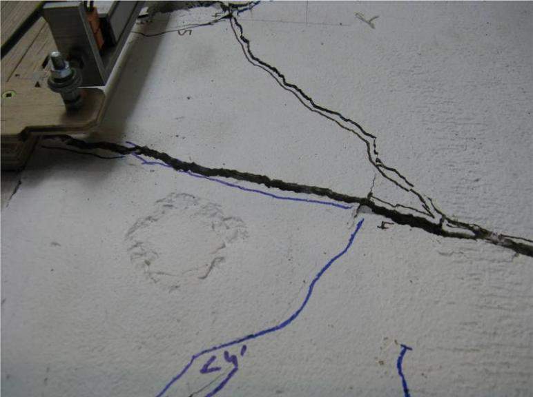
Figure 4.25 – Cracking of the concrete
