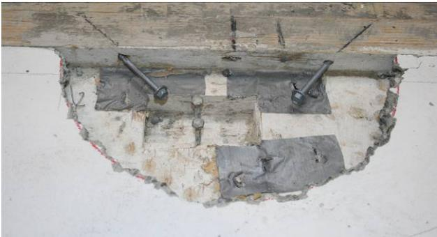
Figure 3.7 – Gap in the concrete which was filled with grout
