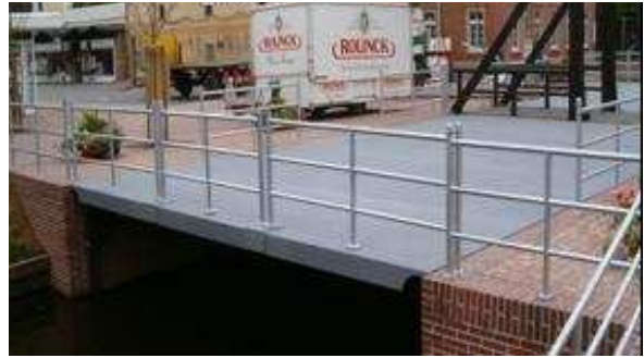
Fig. 2.13. Toepassing I-core paneel in brugdek; Ref. [11]
