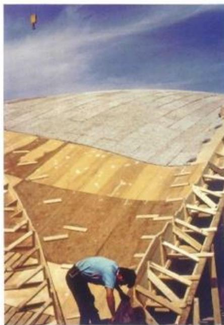
Figure 1.4: Formwork of shell at Heimberg, Switzerland. On top the woodwool panels can be seen. Photo taken from the Journal of the international association for shell and spatial structures (IASS) Vol 52 (2011) No. 3
