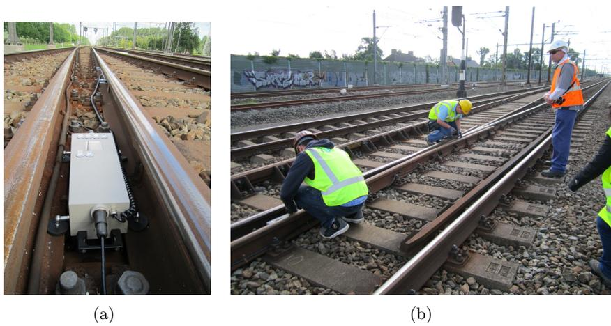
**Figure 8-2:** Installation of ESAH-M device
