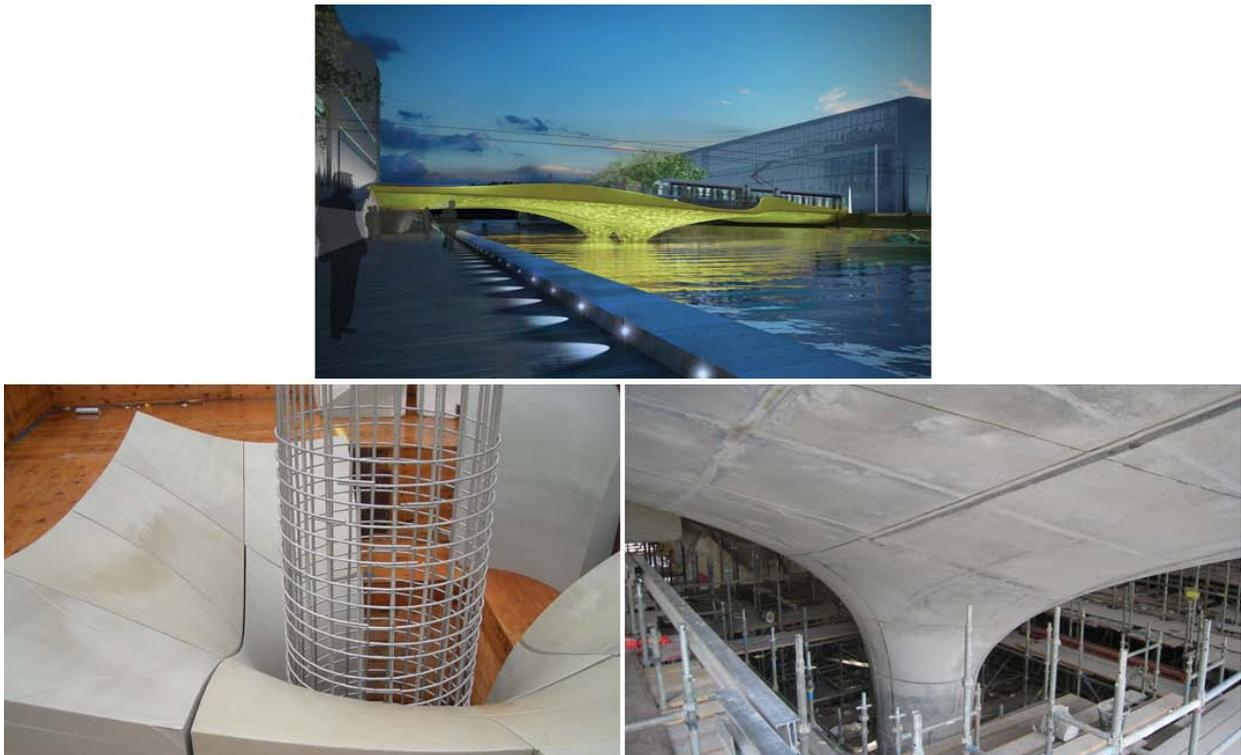
**Figure 8.2.** The Spencer Dock Bridge in Dublin. Bottom-left: The polystyrene mould parts. Bottom-right: The finished section of the bridge ([www.amamdalevetearchitects.com](http://www.amamdalevetearchitects.com);
