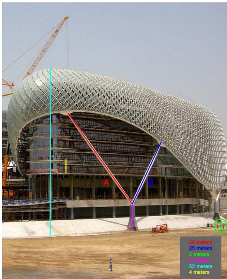
**Figure 3.5.** Rough Dimension of Structure
