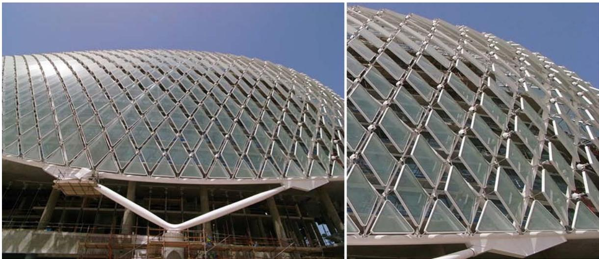
**Figure 3.2.** Diamond shaped panels on Grid shell (Yas-HotelPress Release, 2009).
