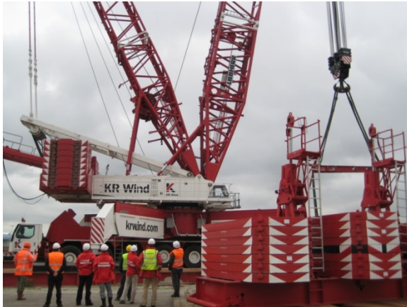
Figure A-14: Application of equipment
