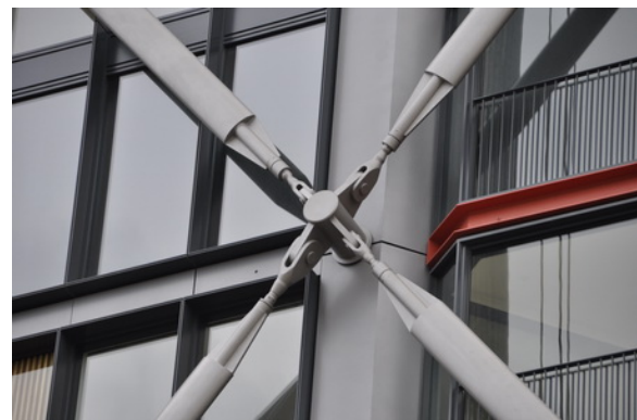
Figure A-4: Bracing system
