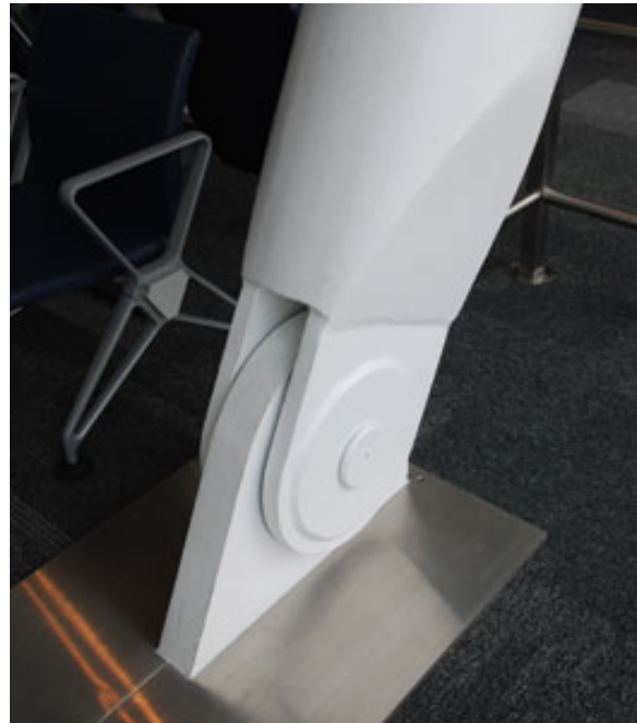
Figure A-6: Finished pinned member
