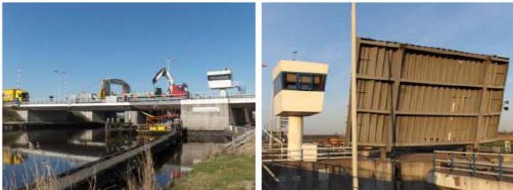
Figure 3.19 Scharsterriijn bridge (fixed part on left side and movable part on the right side) (left); Orthotropic deck of the movable part (right) (Freitas, S.T., et al , [22])
