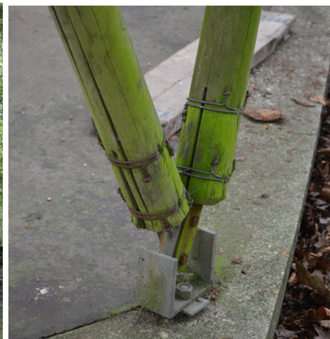
(b) Severe splitting at log ends
