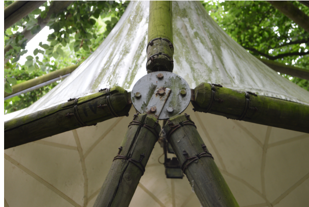
Figure 3.7: Dome hub employed in Geodesic Timber Dome in Botanical Garden Delft
