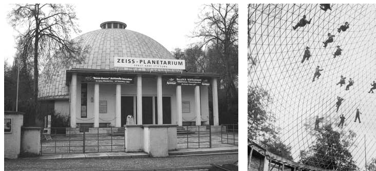
Figure 2.5. Zeiss Planetarium (1925) by Dischinger, Finsterwalder and Bauersfeld, www.structurae.co.uk
