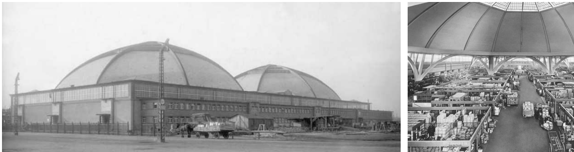
Figure 2.7. Leipzig market hall (1929) by Dischinger and Finsterwalder, www.structurae.co.uk
