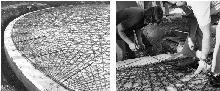
Figure 4.10. Steel spring reinforcement for a BINI Shell structure just before inflation, www.binisystems.com
