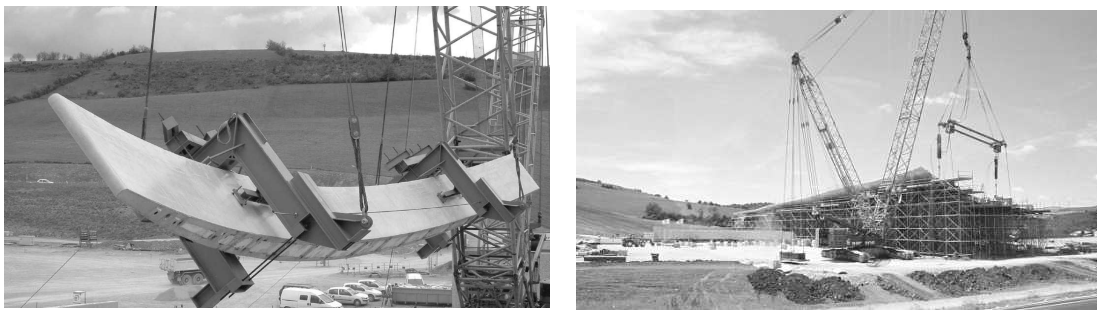
Figure 4.16. Placement of the prefabricated elements on temporary scaffolding of the Millau shell (2005), Servant 2006
