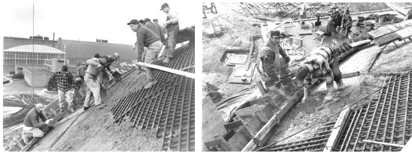
Figure 4.12. The placement of concrete at the Kresge Auditorium (1955), www.arch.e.psu.edu
