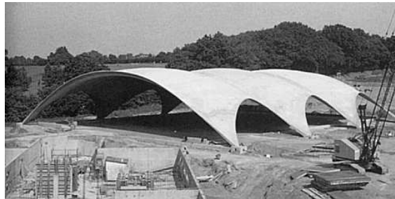
Figure 3.19. The shell as built by Isler for a tennis hall in Dürren (1978)
