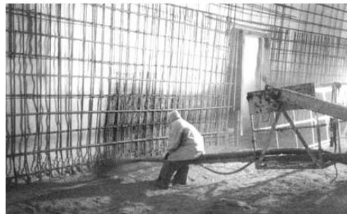
Figure 4.13. Spraying the concrete inside the airform of a Monolithic Dome, www.monolithic.com
