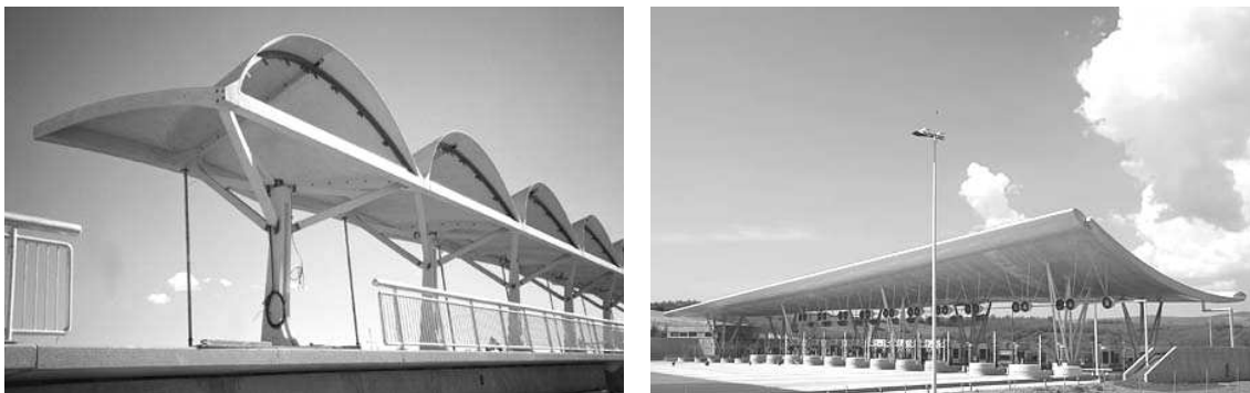
Figure 8.1. Shawnessy LRT Station in Calgary and the Tollgates near Millau, structurae.co.uk
