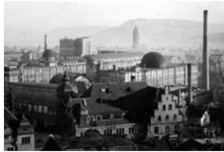
Figure 2.4. The experimental canopy on the Zeiss factory, http://ke.arch.rwth-aachen.de
