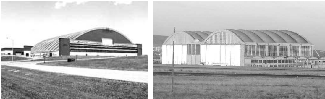
Figure 2.23. Airplane hangar (1949) Limestone, Weingardt 2007, and the Marignane hangar (1952), www.structure.co.uk
