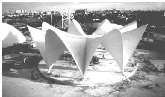
Figure 3.25. Shell l'Oceanografic in Valencia constructed from as well fibres as a reinforcement mesh, www.structurae.co.uk
