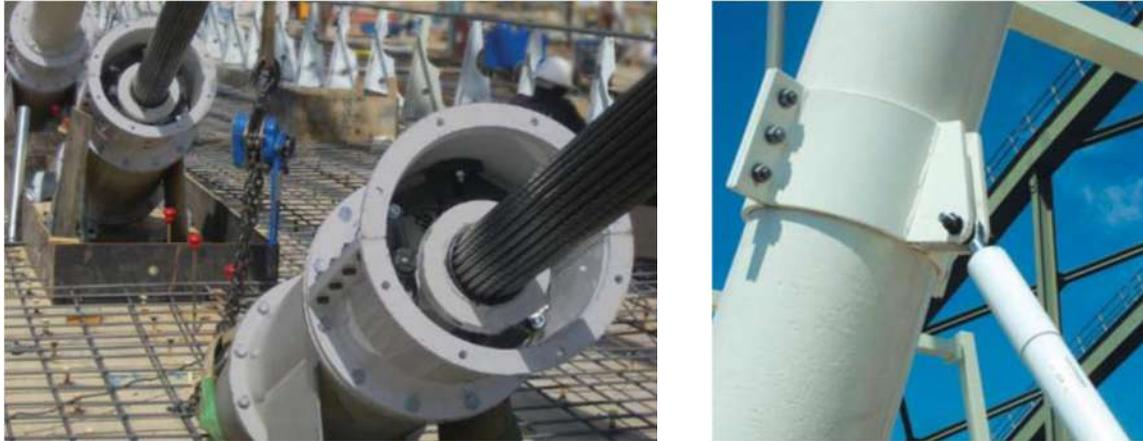
Figure 35: Dampers in anchorage of parallel wire cable (left), externally attached damper (right)
