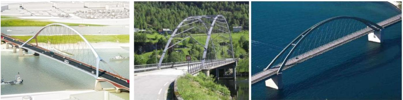
Figure 10: Single arch, double arch, basket handle arch (left to right: De oversteek bridge, Bolstadstraumen bridge, Fehmarnsund bridge)
