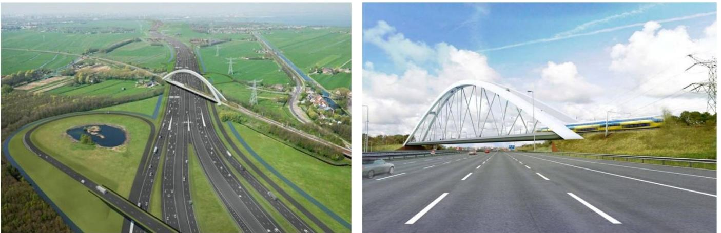
**Figure 1: Artist impressions of the arch bridge with diagonal hanger arrangement that will be built to cross the widened A1 highway (10 lanes)**
