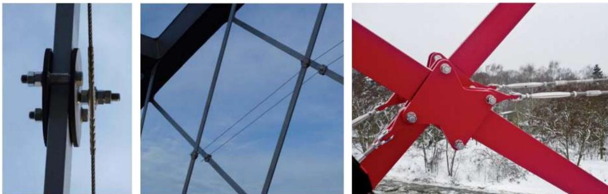
**Figure 34: Stabilizing cables**
