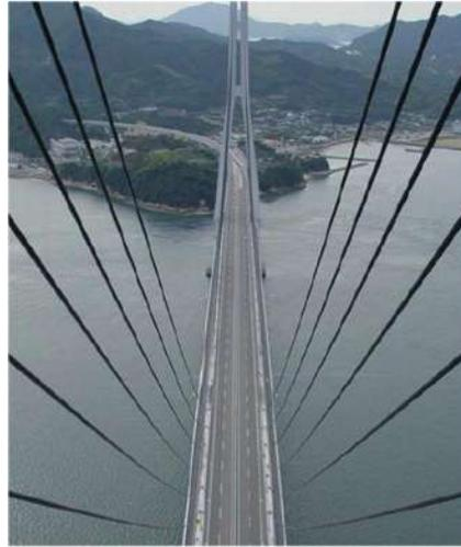
Figure 136: Hangers of a cable stayed bridge, the catenary effect becomes visible
