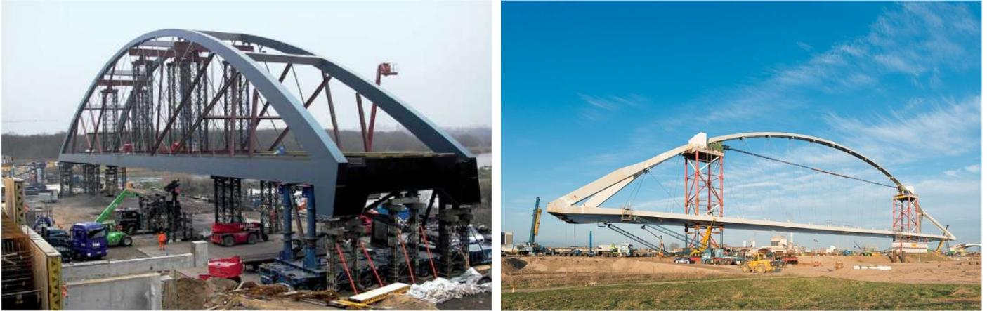
Figure 42: left: bridge with supported hangers to prevent buckling, right: Oversteek bridge ready for transport
