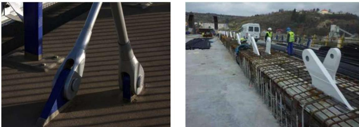
Figure 15: Examples of concrete main girders and hanger connections (left: Trinec-Baliny Road bridge, right: Troja bridge in Prague)
