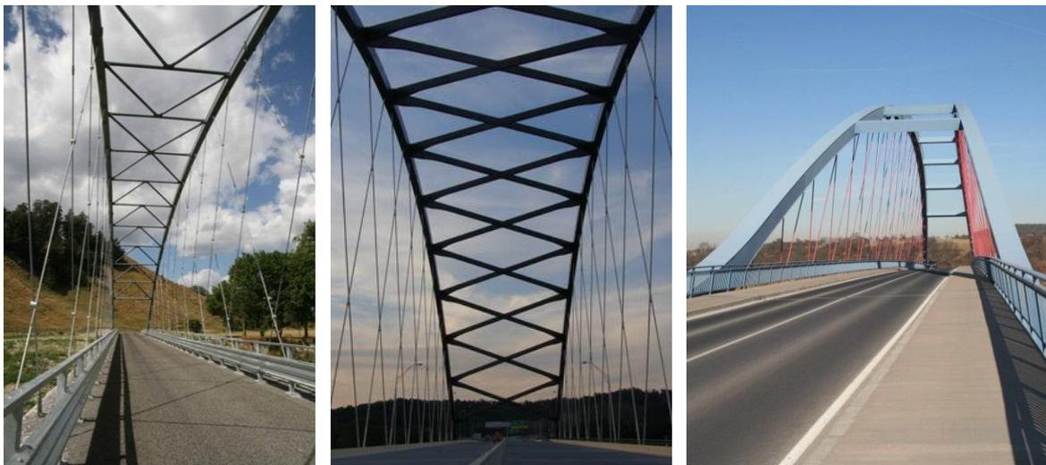
Figure 13: lateral bracing (left: K-truss, middle: diamond truss, right: Vierendeel truss)
