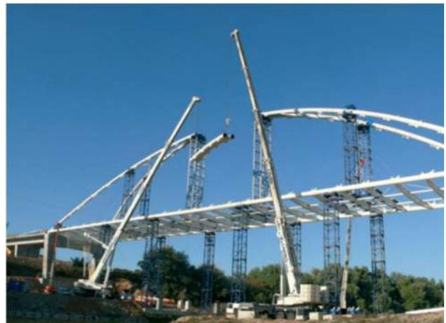
Figure 38: Final assembly of the arch, left: Oversteek bridge, right: Palma del Rio bridge
