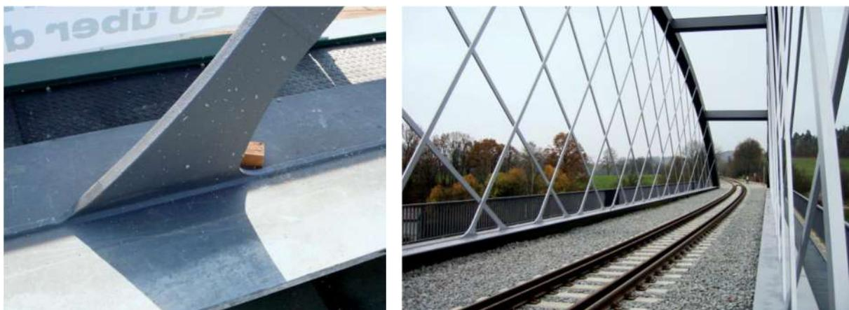
Figure 21: Flat steel hangers (left: unknown bridge, right: Rosenbachtal railway bridge)
