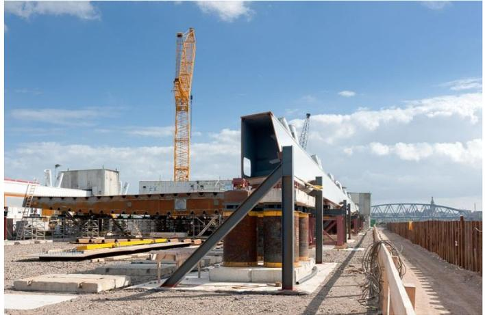
Figure 37: left: temporary support of bridge constructed at final construction site (Palma del Rio bridge), right: temporary support of main girder (Oversteek bridge)
