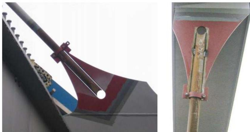
**Figure 40: left: temporary hanger/ main girder connection, right: arch/ main girder connection**
