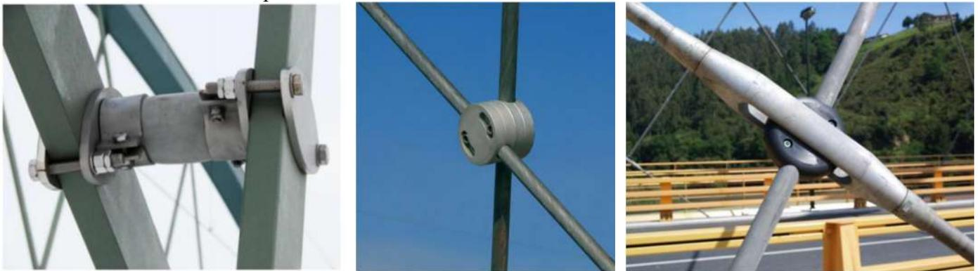
**Figure 33: Intermediate hanger coupling without damping**
