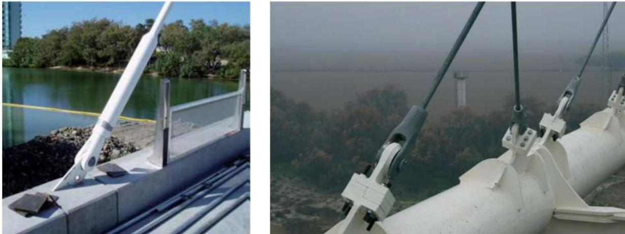
**Figure 23: Fork connectors for cable systems, left: Freyssinet fork connector for parallel strand cable, middle: fork connector for spiral strand**
