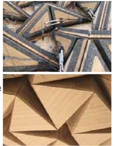
Image 3.23. Actuation and suspension details of Resonant Chamber as seen from above (top) and folding surface deformation from below (bottom) (image courtesy of Thün 2012).
