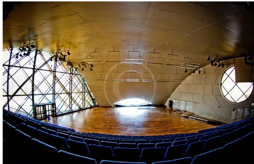
Image 1.5. Form and system follow acoustic functions: ceiling shape is an optimal but non adaptive system (Ravello Auditorium, Oscar Niemeyer desing)
