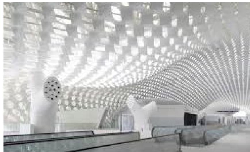
Image 2.40. Shenzhen Airport, Massimiliano and Doriana Fuksas design. An example of functional integration of structure and environmental control executed by 2D-rigid panels.
