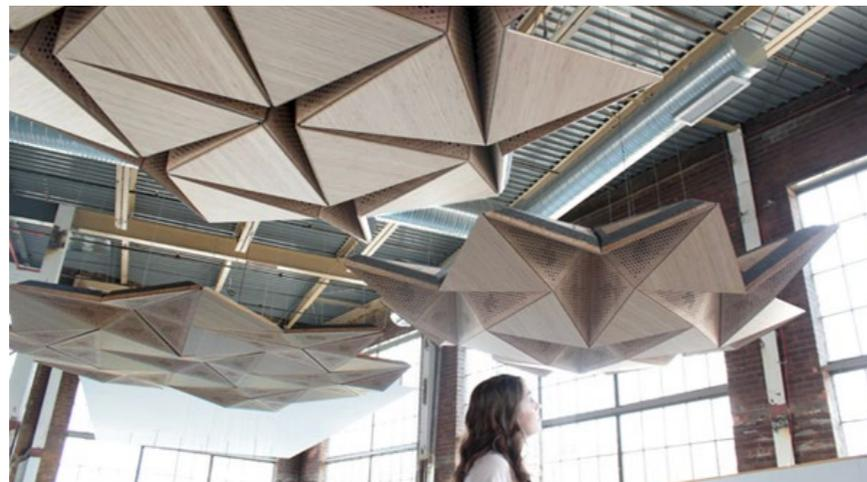
Image 2.11. Resonant Chamber, prototypes for an adaptive acoustic ceiling (image courtesy of eVolo.us).
