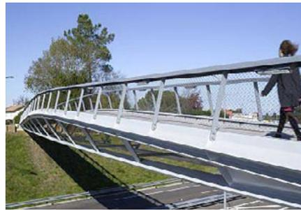
Image 2.57. A stress-ribbon rigid deck together with two further ties compose this lightweight bridge. RFR design.
