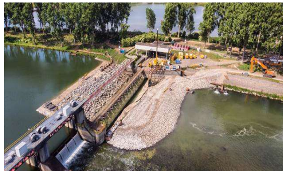
Figure 2.13: reparation of weir Linne [52]
