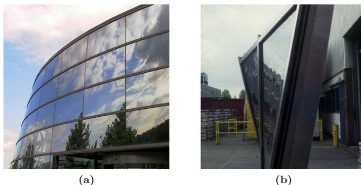
**Figure 1.5:** (a) Glass facade supported by frames, Ford Research Center (Carbonell Figueras) (b) Frame support (Reynolds)
