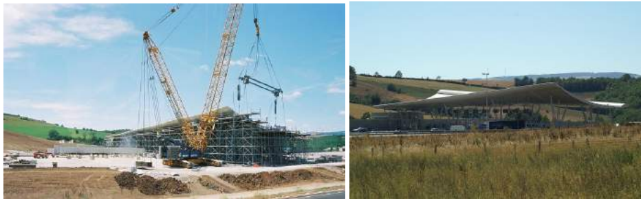
Figure 2.6: (a) Construction of the roof (b) Millau toll station, [3]
