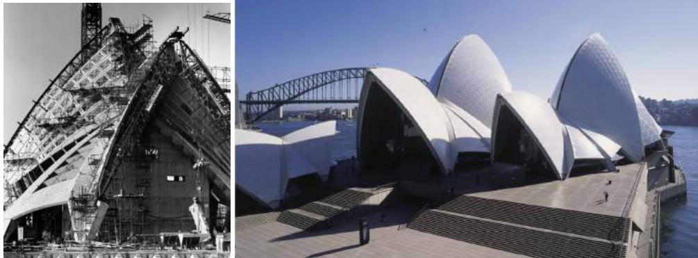
Figure 2.3: (a) Construction of the shells (b) Sydney Opera House
