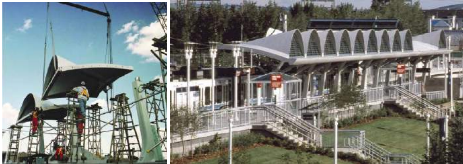
Figure 2.5: (a) Construction of the shell (b) The Shawnessy LRT station
